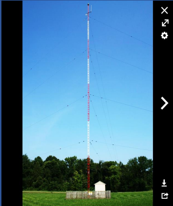
A typical mast radiator and antenna tuning hut of an AM radio station in ...
